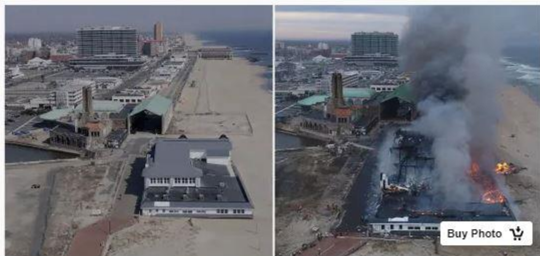
The pavilion at the north end of the Ocean Grove boardwalk is shown (left) on March 20, 2019, and then (right) as a massive fire consumed the structure Saturday, April 13, 2019. (Photo: Thomas P. Costello, Tariq Zehawi & Danielle Parhizkaran)
