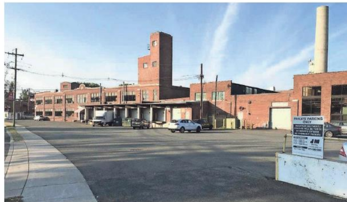
An Industrial zone on Wagaraw Road in Fair Lawn. SHAYLAH BROWN/NORTHJERSEY.COM
